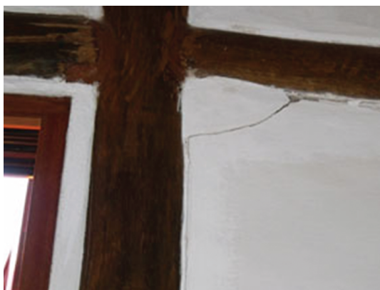
Figura 13. Pilar B8 e parede interna com fissura recente. Figure 13. Column B8 and the inner wall with recent cleft.
